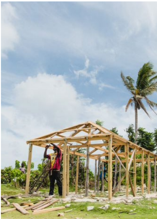
A Technician constructs a demonstration house frame. Photo: CRS
