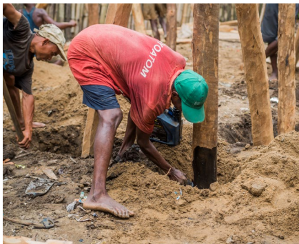
Hard woods are used for posts, dug 1 meter into the ground, and protected with a coating of motor oil.
