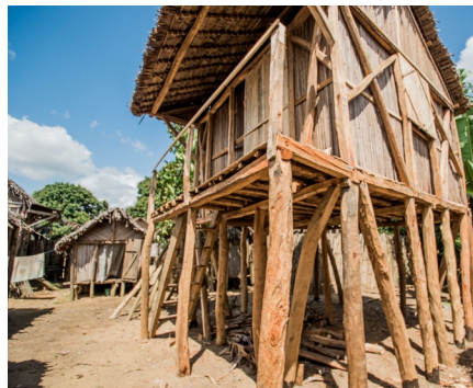
The stilts are reinforced with cross-bars on all sides.
