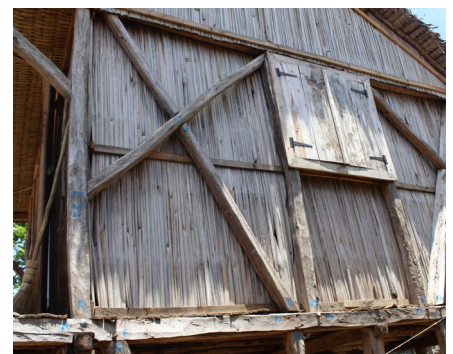
Diagonal bracing in all wall angles.
