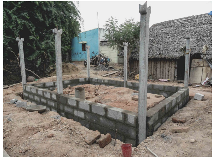
A plinth protection wall reduces erosion during flooding
