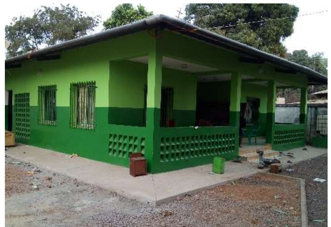
Housing facilities (back and left view), Kankan, after.
