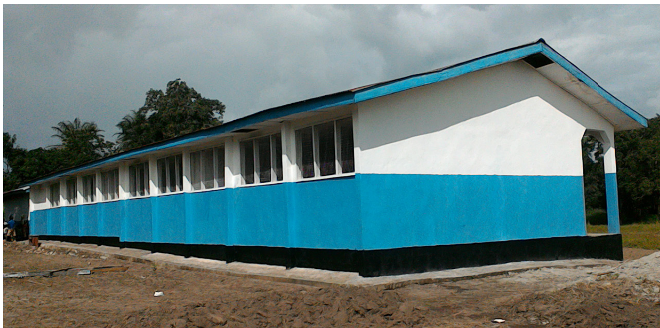
Completed school block. Photo: CRS
