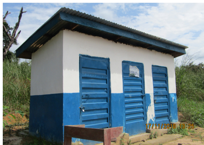
VIP Latrine after completion. Photo: CRS
