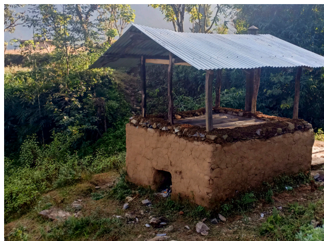
A large cardamom double dryer drum established by farmer groups at Aaruarbang # 7 Aapric with project support. This improved drying technology helps reduce post-harvest losses and increases the quality of large cardamom. [Photo by CRS Staff]
