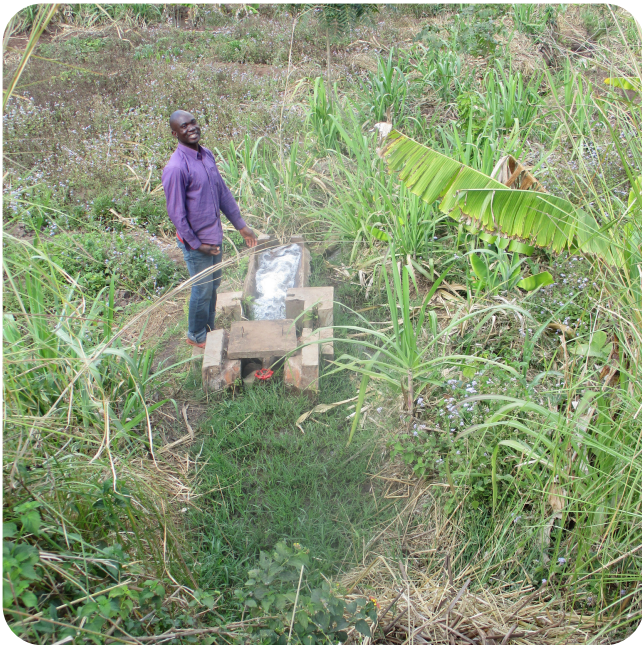
Figure 2: A WMC member poses beside the new irrigation gate valve that the community replaced last year when the old one broke.
