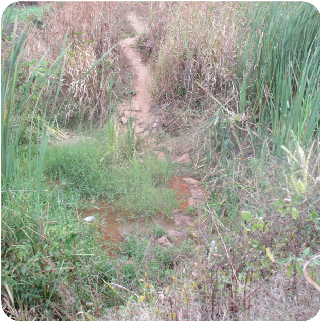
Figure 2: During heavy rains, this earthen constructed weir was washed away.
