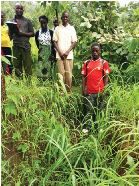
Photo 1. A forest WAT constructed in 2001, Lingoni, showing man in red at the bottom of the trench and man in yellow at top.
