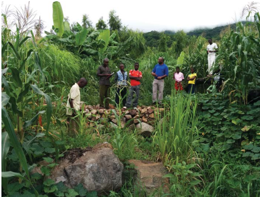
Photo 4. Members of the Watershed Committee standing on a large (about 12-m) check dam, which has reclaimed a barren gully, Lingoni.
